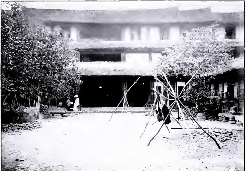
FORTIFIED DWELLING : YUNGCHUN VALLEY (Interior).
